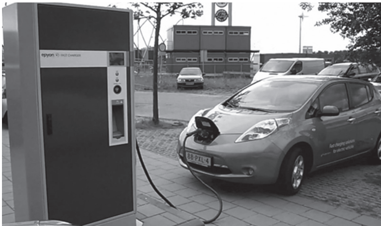
An Epyon/ABB DC fast charging station with a Nissan Leaf being charged
