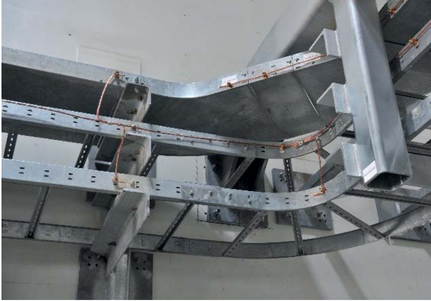
Figure 2. Meshed Bonding Network (© A.P.J. van Deursen)
