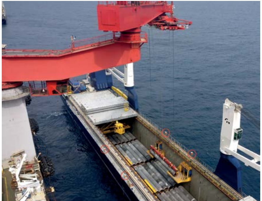
Figure 1. The spreader bar picking up a pipe joint
