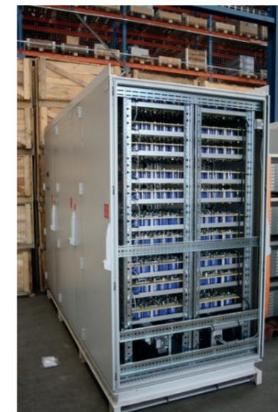
Figure 1. Super capacitor-based energy storage.
