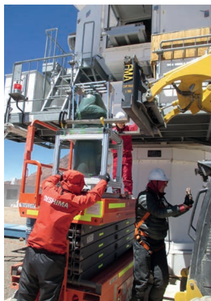
Figure 4. Installation of the DESHIMA cryostat (protected in a plastic bag) to the ASTE cabin.
