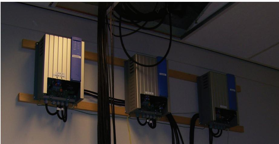
Figure 3: The invertors from the solar panels on the roof
