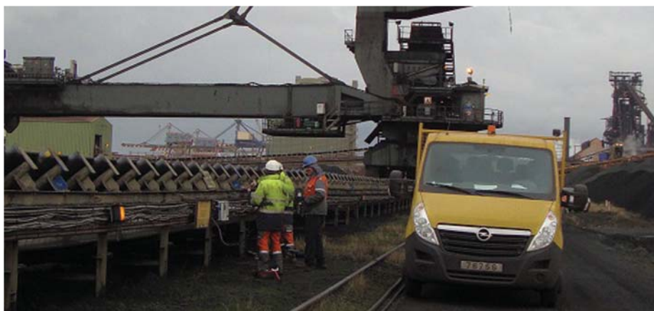
Figure 3: Idler rolls inspection
