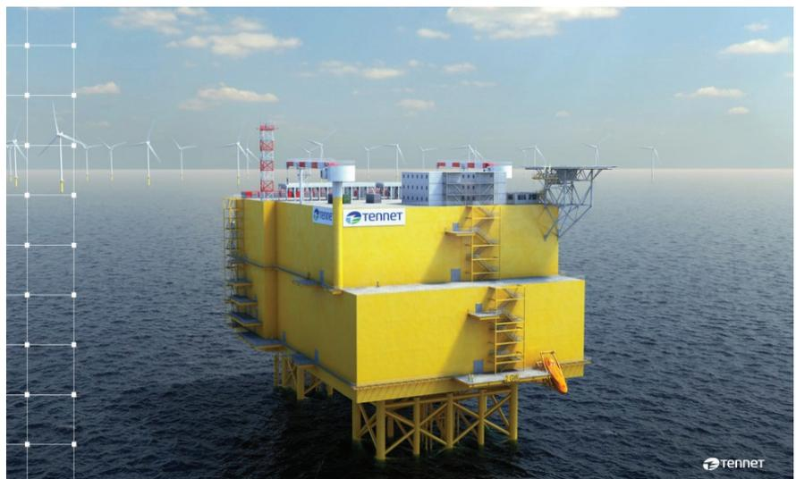
**Figure 1.** 2000 MW Voltage Source High Voltage Direct Current converter station connecting future large offshore wind power plants
