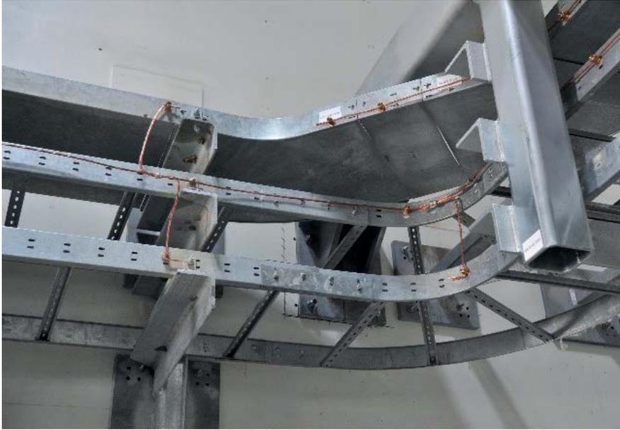
*Figure 2. Meshed Bonding Network (© A.P.J. van Deursen)*
