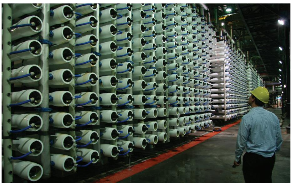
An array of membranes used for the desalination of water
